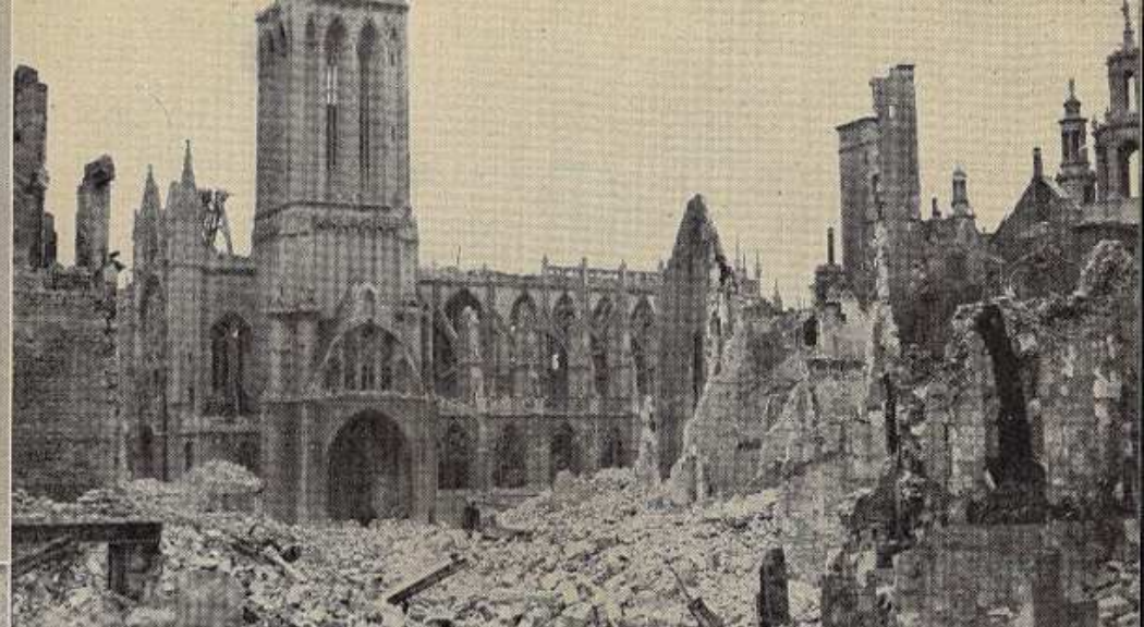
CAEN - Ruined main street in which stands the damaged XIVth-century church of St. Pierre.
