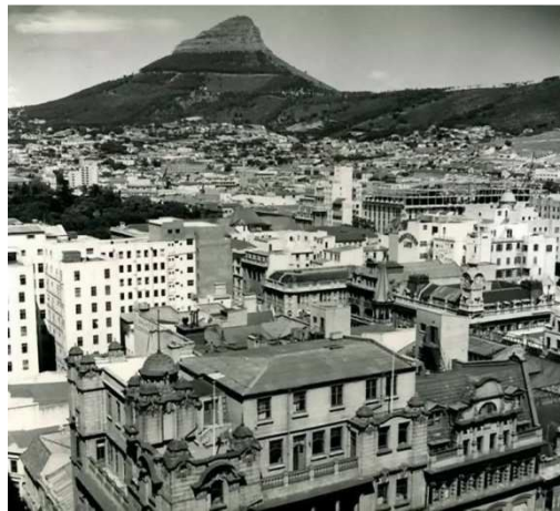
Cape Town – 1942 (cape-town.photos)
